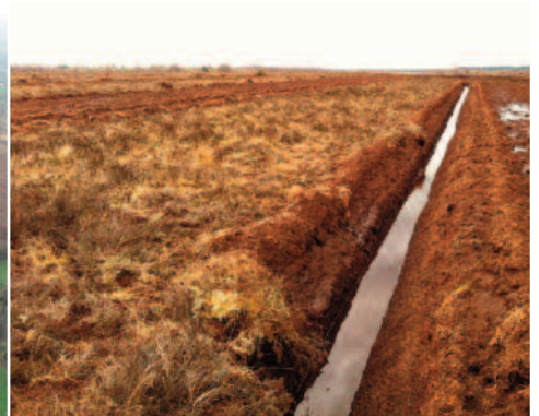
Figure 5: Surface view of Cloonroosk bog showing drain and the disruption to the bog surface through the spraying of material from the drain onto the living peat forming moss layer.
